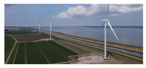
Kroningswind is an onshore windfarm on the island of Goeree-Overflakkee in South Holland, located on farmland between the towns of Stellendam and Middelharnis. The windfarm consists of 19 Vestas turbines with a total capacity of approximately 80 MW.
