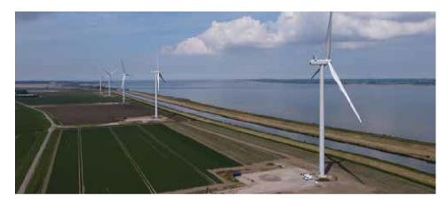
Kroningswind is an onshore windfarm on the island of Goeree-Overflakkee in South Holland, located on farmland between the towns of Stellendam and Middelharnis. The windfarm consists of 19 Vestas turbines with a total capacity of approximately 80 MW,
