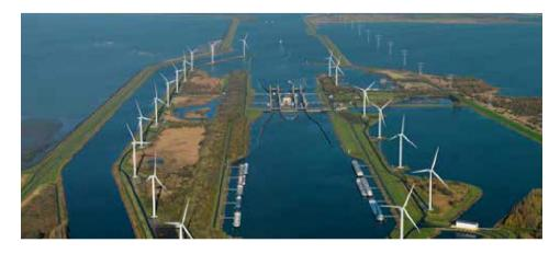
Kreekraksluis windfarm is an onshore windfarm on and near the Kreekraksluizen locks in the Scheldt-Rhine Canal in the municipality of Reimerswaal in the Dutch province of Zeeland, The windfarm has 16 Nordex turbines with a total capacity of approximately 40MW,
