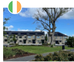
TINC ups its stake in Irish Social Housing PPP to 100% October 2022
